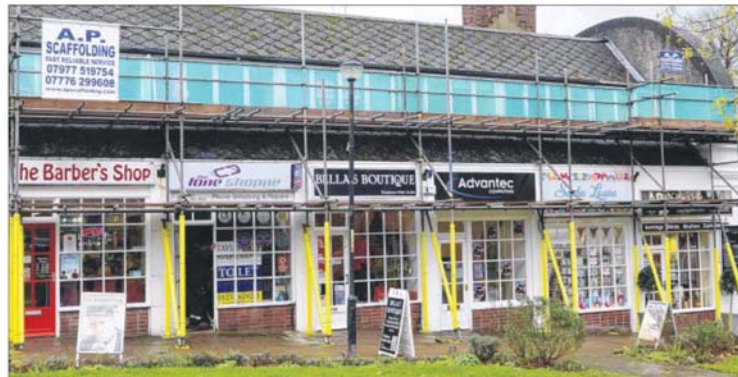
Scaffolding around the businesses at The Fairings
