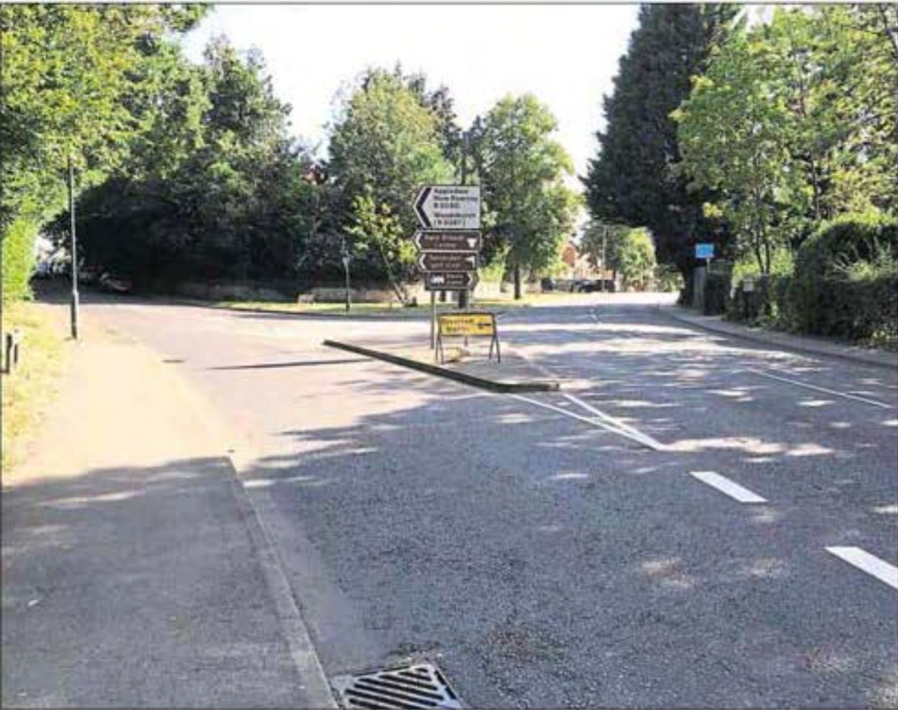
The junction with Ashford Road and Beacon Oak Road
